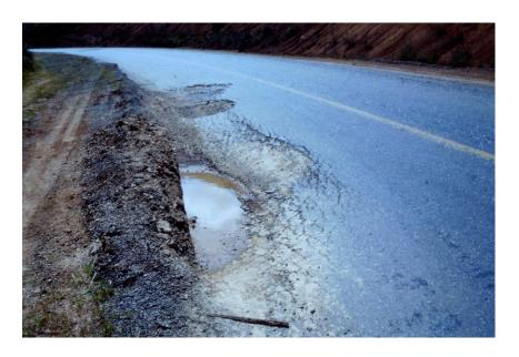
Poor pavement drainage arrangements and lack of timely maintenance. This was exacerbated by uncontrolled overloading of trucks.
