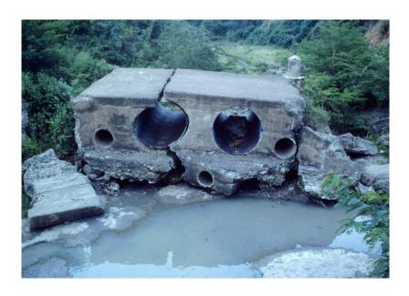
Where do you start?? It seems that attempts to 'improve' the structure have been made at various times – unsuccessfully! Design shortcoming indicate lack of peak flow capacity, lack of substructure and side seepage measures. There were also no restraints to prevent vehicles falling off into the watercourse.
