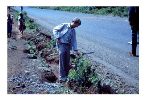
The road shoulder has been severely eroded by rainwater. The cause is inadequate drainage measures at the design/construction stage and failure to maintain the shoulder. Obviously a highly dangerous situation, particularly at night.
