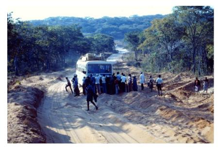
The road surface consists of the in-situ, generally single sized particle sand with no fines able to bind the material together. Any traffic displaces the material and vehicles get bogged down. The solution would have been to stabilise the material or cover it with a more robust surface material, unfortunately both expensive solutions.
