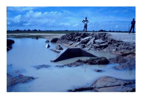
The culvert was substantially undersized and suffered from overtopping, support and backfill erosion, and foundation failure (absence of anti-seepage measures).
