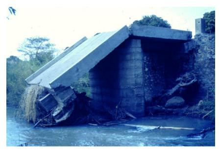
This image was taken in the dry season. The structure was obviously not designed long enough to bridge wet season flows leading to erosion of the abutment foundation and failure.
