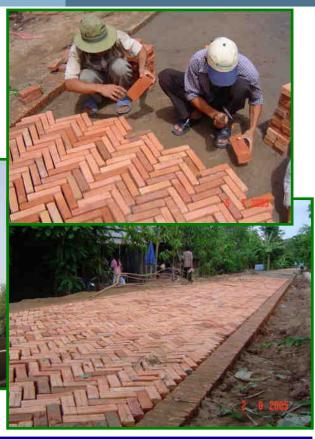
Burnt Clay Brick paving can be an important option in areas lacking hard stone resources, for example in delta regions. The clay can be fired to high quality bricks using small scale kilns and renewable energy sources, such as waste rice husk. Materials haulage can be minimized and local employment created in brick production for roads and building construction.
